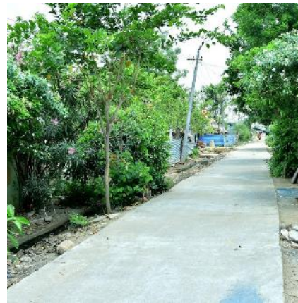
Cement Concrete Road- Enkoor Mandal, Khammam District
