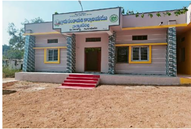
Grampanchayat Building, Kyatanpalle GP, Damaragindda Mandal, Narayanpet District
