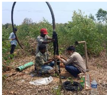
Flushing and Repair of Borewell Works at Bhadradi District
