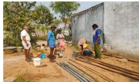
Hand pump repair at vilochavaram , Manthani(M)
