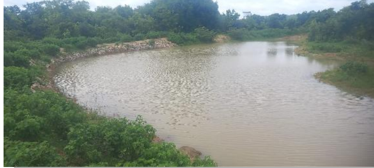
Percolation Tank, Varni Project, Mallaram MWS,
