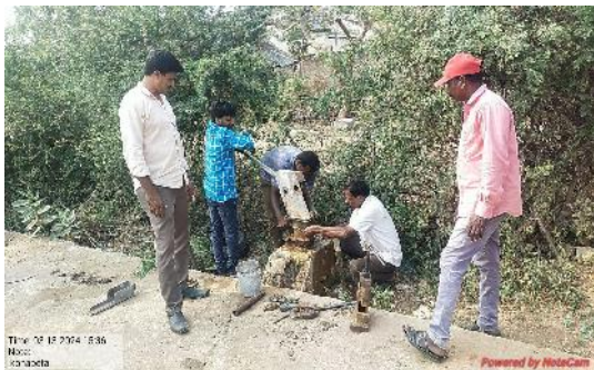
Hand pump Repair at Rajaka Bazar of kothapeta , Bayyaram(M)
